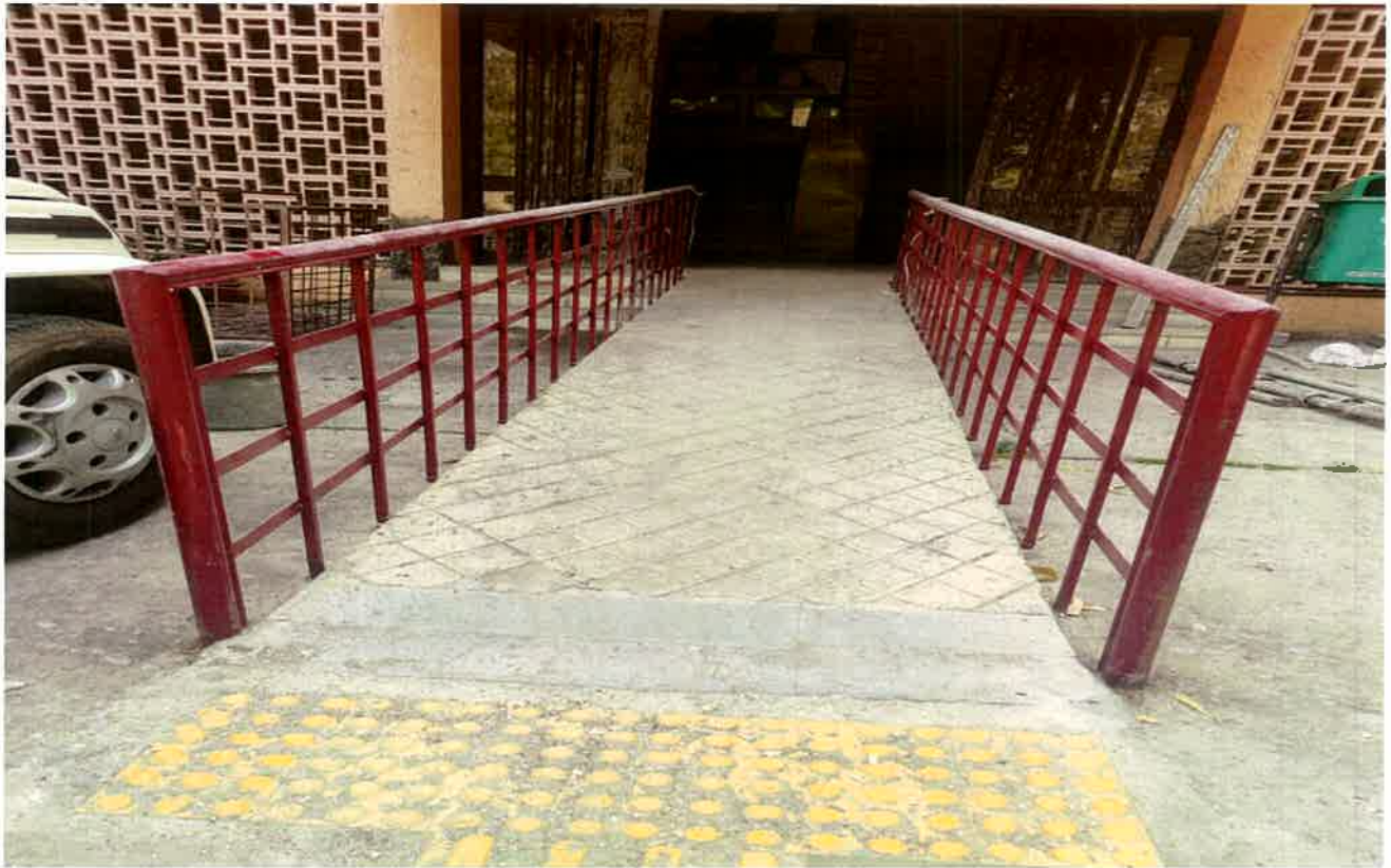
Ramp constructed around the campus to help the differently abled students
